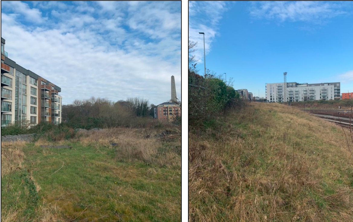
Figure 20-31 (Left photo) View North of the Compound/ Attenuation Area to the West of the Mainline Track. (Right photo) and View West towards the Site of the Island Bridge Substation
